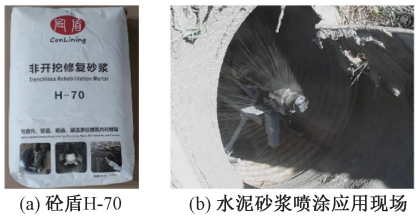
图 7 国产纤维增强高性能复合水泥喷涂砂浆(砼盾 H-70)及其应用现场 [33] Figure 7 Domestic fiber-reinforced high-performance composite cement spray mortar (Concrete Shield H-70) and its application site [33]
