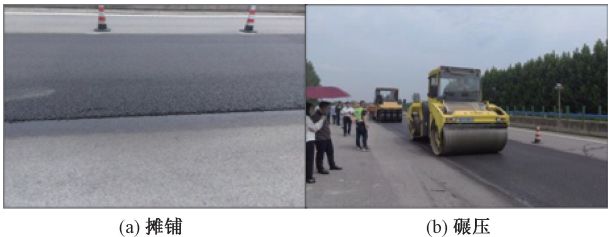
图 8 路面摊铺与碾压 Figure 8 Pavement spreading and rolling
